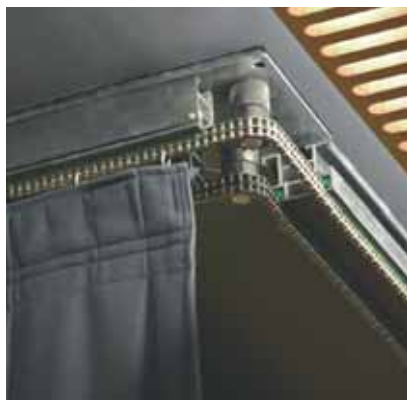
Tracking a curtain into a pocket behind the walls of Hall One.
